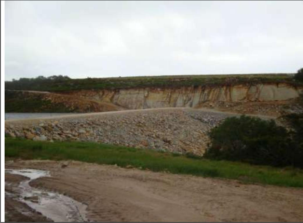
Downstream face protected with rip-rap with spillway excavation in the background.
