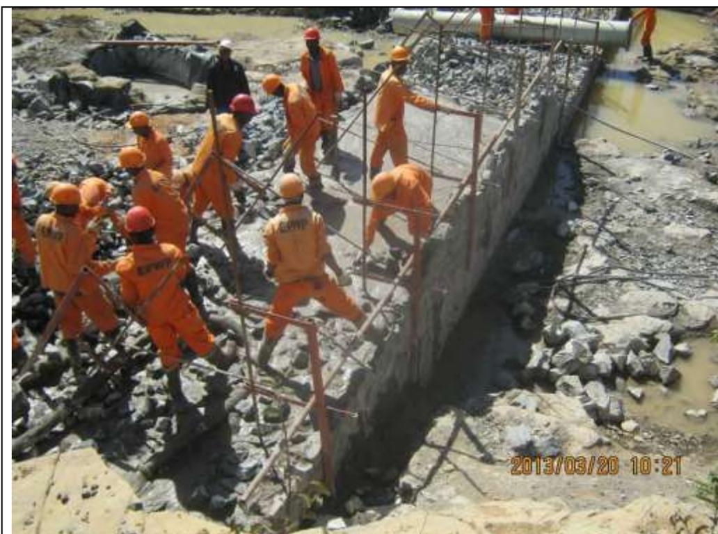
Pouring concrete on the tail pond toe in progress.
