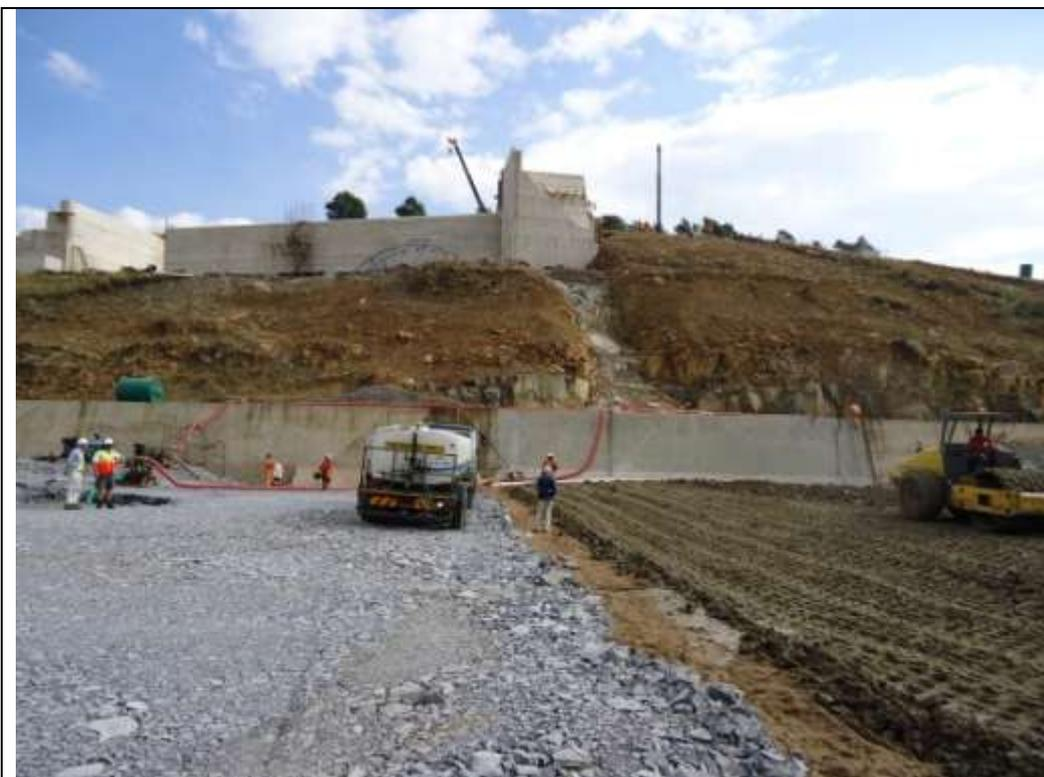
Construction of the rockfill dam with clay core underway, after repair of coffer wall.
