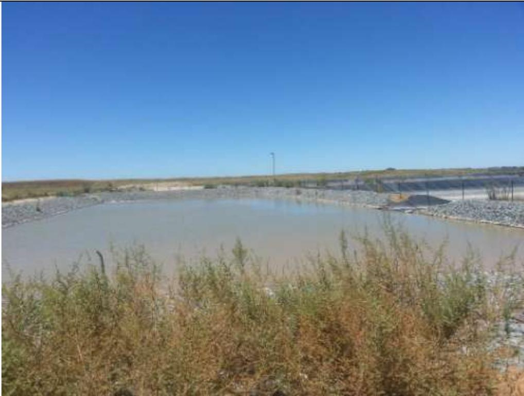
Return water dam. Filtered water is transported through pipes to existing tailings dams to make more sludge for gold processing.
