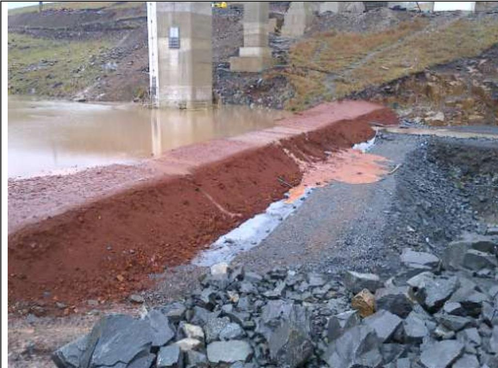
Photo shows coffer wall upstream of main dam wall just before being overtopped.
