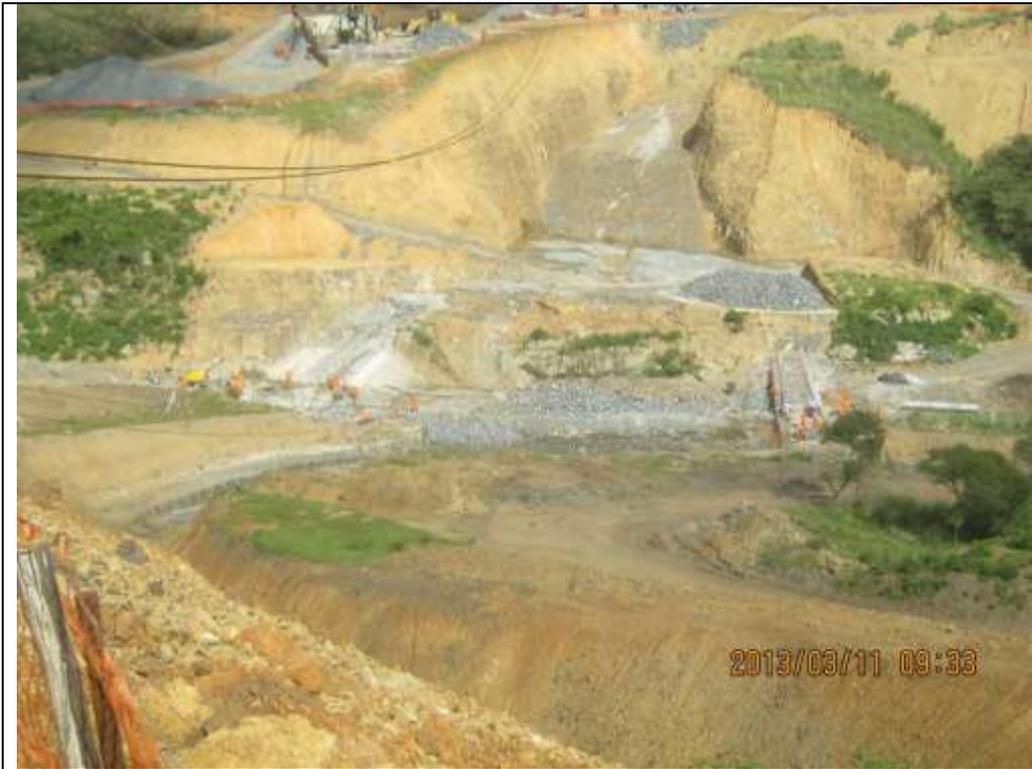
Excavation for a new rubble masonry concrete arch dam.
