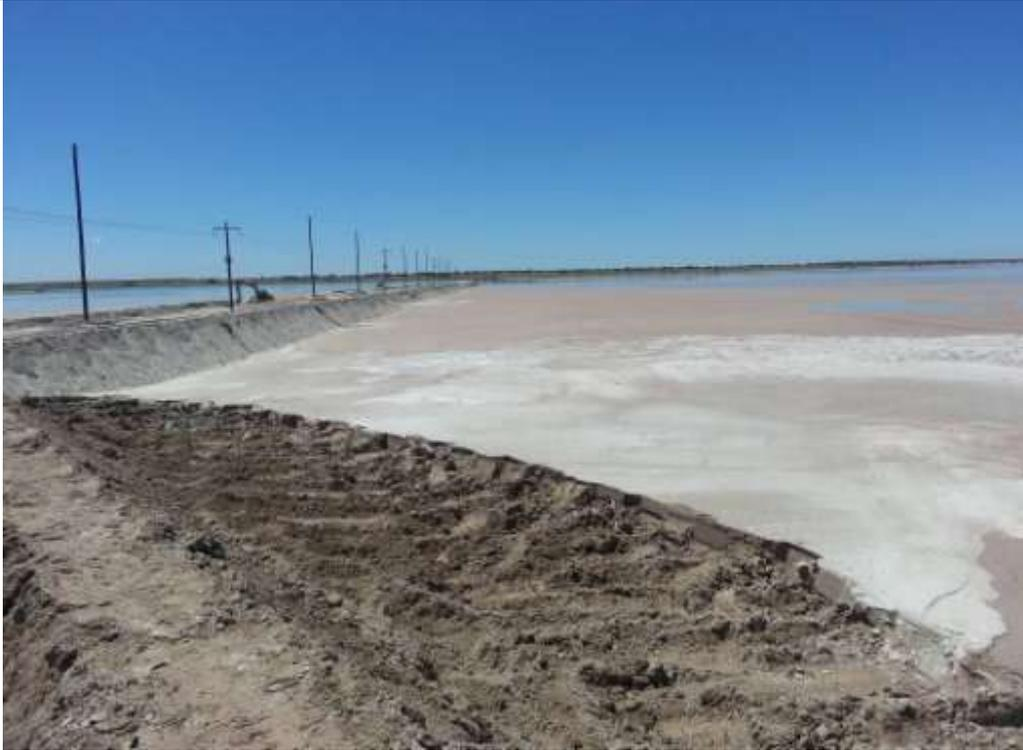
About 1000m<sup>3</sup>/hr of sludge is transported from existing/ decommissioned tailings dam to a pumpstation onto the Chemwes Kareerand Tailings Mega Dam and deposited via cyclones.
