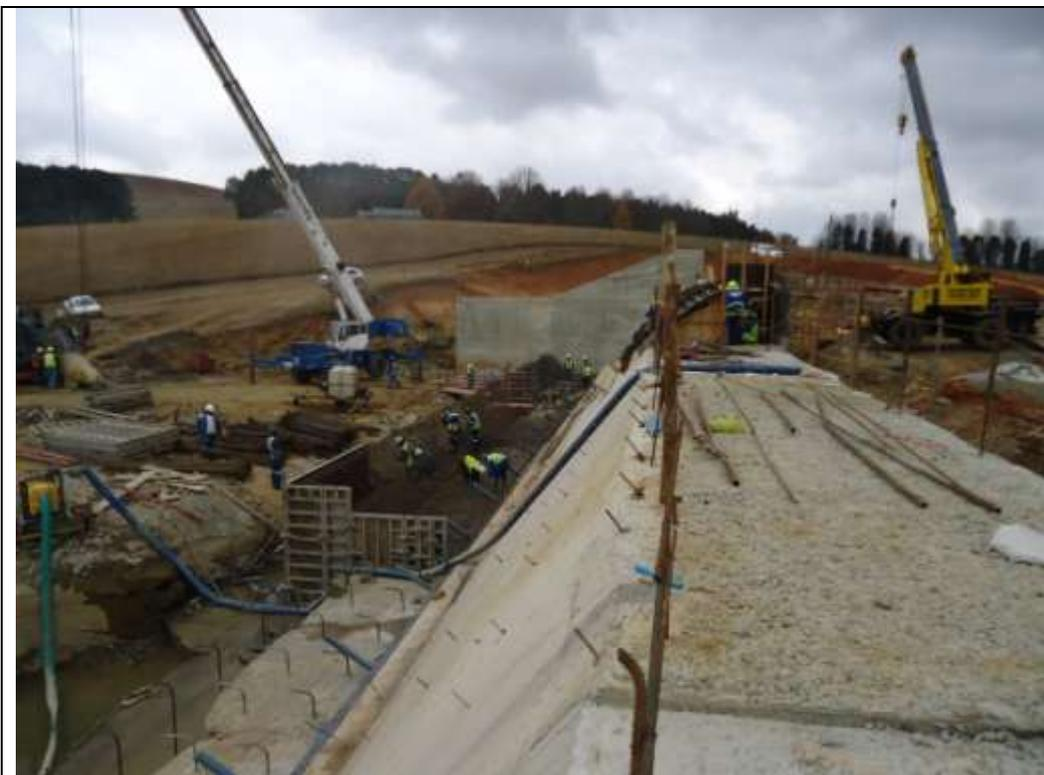
New Fish Barrier Weir being built just upstream of waterfall in Mooi River to replace natural fish barrier.
