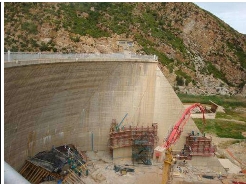
Concrete delivery into a lift in the left buttress.
