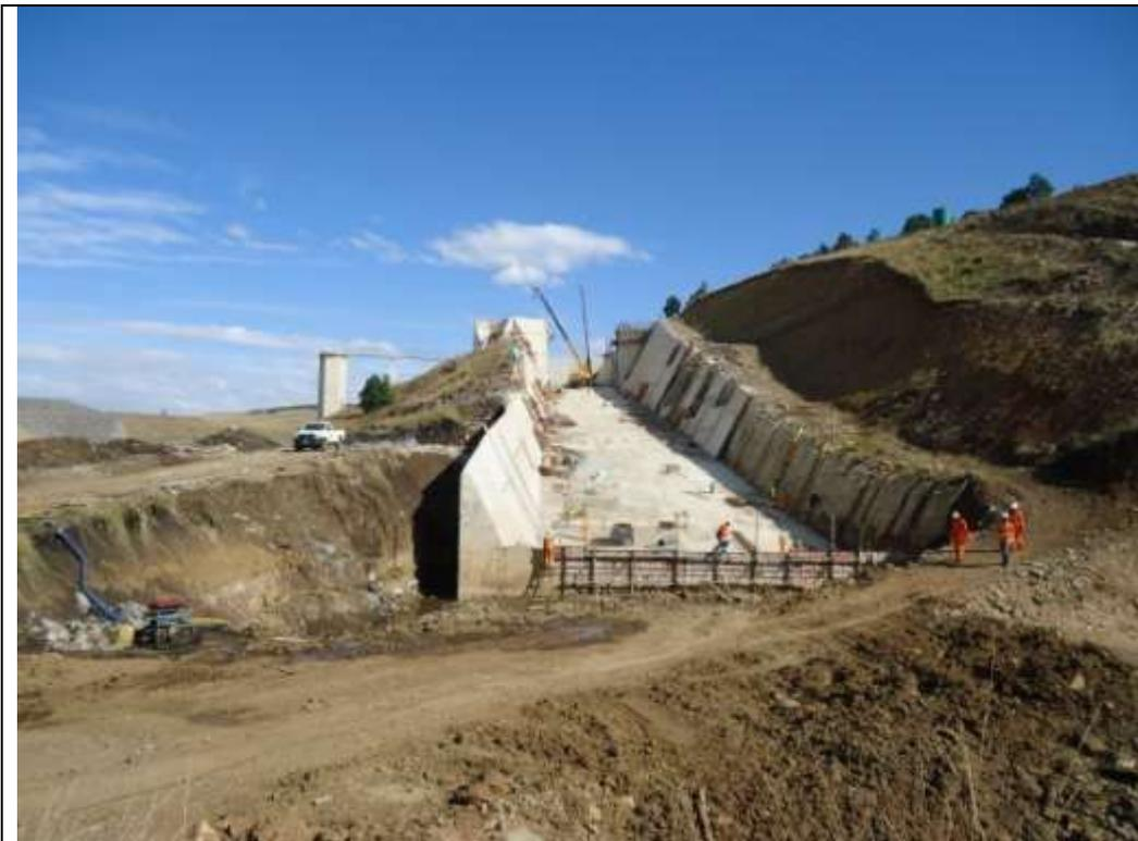
Picture of downstream part of side-channel spillway. Soil nails were used to anchor side walls.
