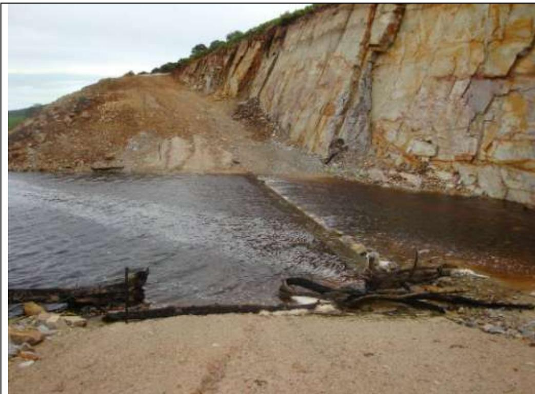
Spillway in operation showing first sill on the upstream side..
