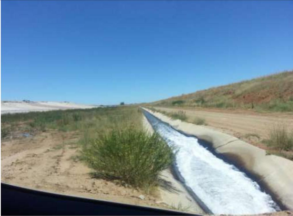
Canal carrying decanted water. About 2000m<sup>3</sup>/hr is continually moving through this system.
