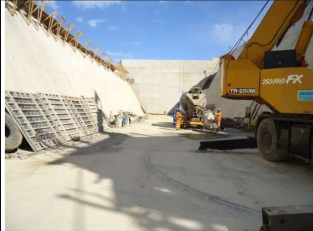
Side-channel spillway under construction.
