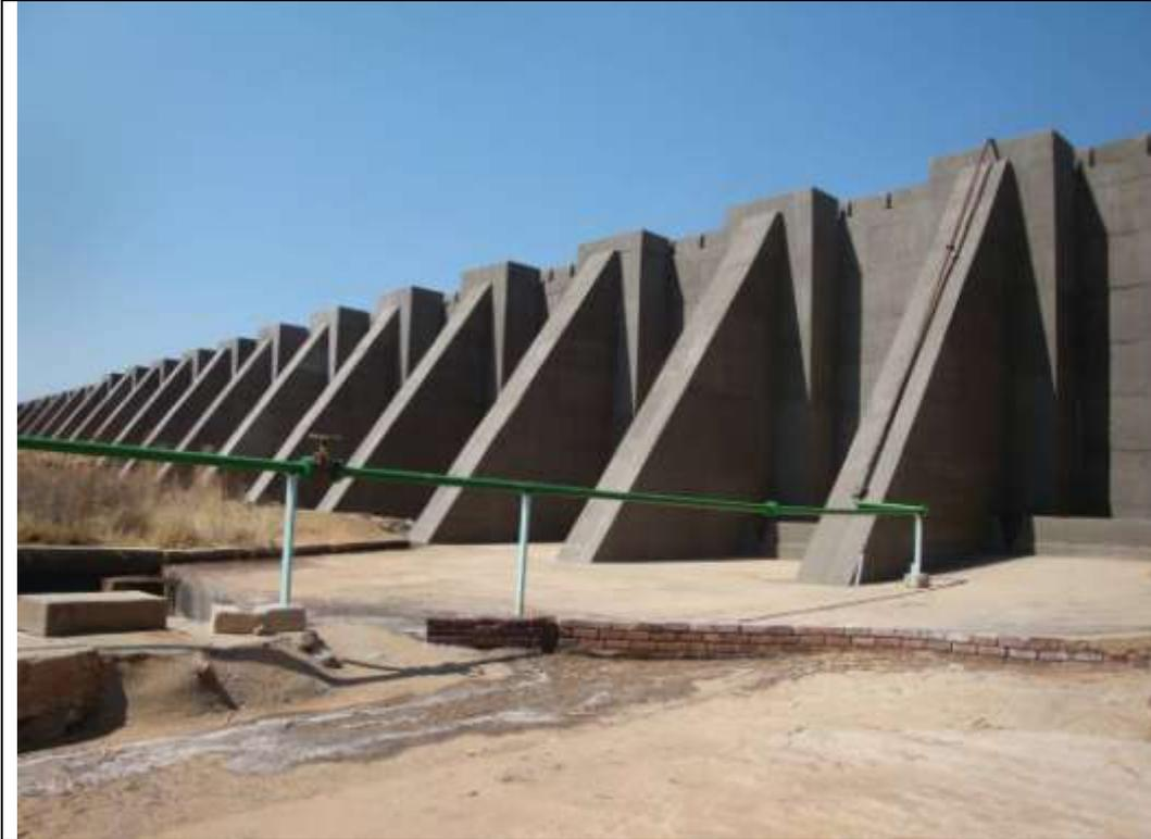
Completion of rehabilitated wall on downstream face of Chloorkop North Dam.
