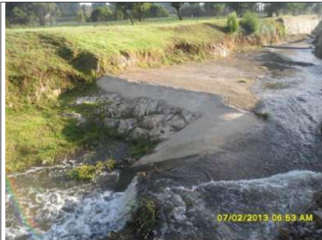
AFTER: Repair on chute and gabion basket retaining wall.
