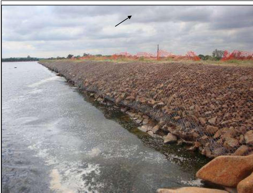
View of replaced rip rap on upstream slope from west side bank.
