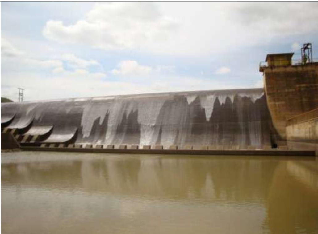
Although the water level was below full supply level, it was spilling slightly on 7 November 2012 due to windy conditions.
